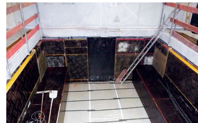
Foundation isolation using RLA 390-14 type belted bellows
