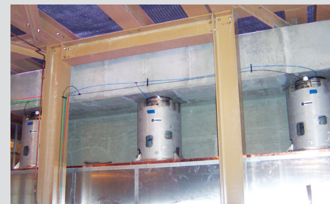
Measuring machine foundation
