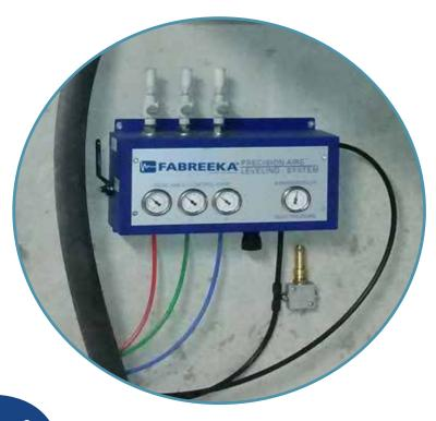
Before the isolation system was installed, engineers at Fabreeka conducted a prestudy to test the dynamic values of the isolation system such as natural frequencies, damping, and vibration values. In addition to the installation of the isolators on the designated hardpoints (shown middle right) a control panel (shown bottom left) was installed which controls the pressure gage.
