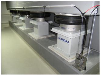
Achieving low frequency isolation with 10 RLAtype pneumatic isolators engineered by Fabreeka for a hydropuls test rig for German sports cars under a 7 by 5 m surface area with a concrete mass of 220 t.
