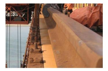
Maintenance workers replace steel plates with CR2-3 rail pad under rails of an unloader crane to reduce wear and vibration.
