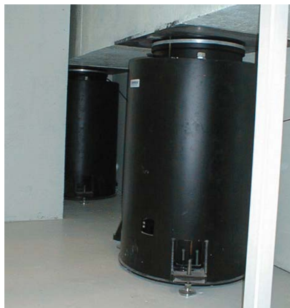
Pneumatic isolators with lifting capacities of up to 120,000 lbs each are used to provide low frequency isolation for large concrete reaction masses (foundations). The isolators shown above are 72" (1,830 mm) in height and have vertical and horizontal natural frequencies of 0.7 and 0.5 Hz respectively.
