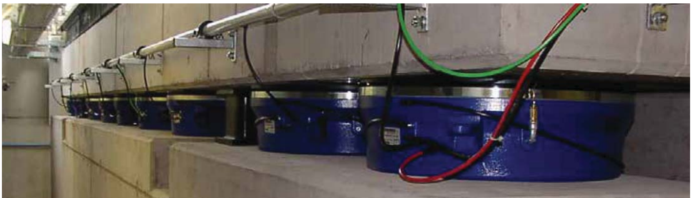
Fabreeka PAL type low frequency, pneumatic isolators support and isolate a foundation having moderate displacement.
