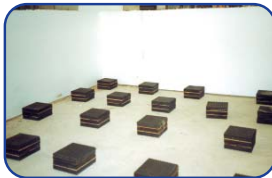
Elastomeric isolators and forming installed on pit floor prior to concrete pour.
