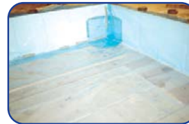
Elastomeric isolators and forming installed on pit floor prior to concrete pour.
