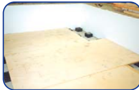
Elastomeric isolators and forming installed on pit floor prior to concrete pour.
