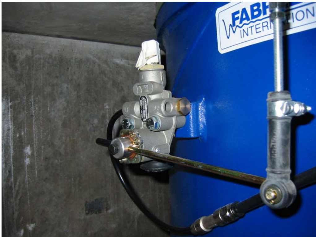
Sixty-six (66) PAL 1000 pneumatic isolators support the first and second floors of the wafer fabrication facility. Each isolator supports 120,000 lbs and has a vertical and horizontal natural frequency of 1.5 Hz.
