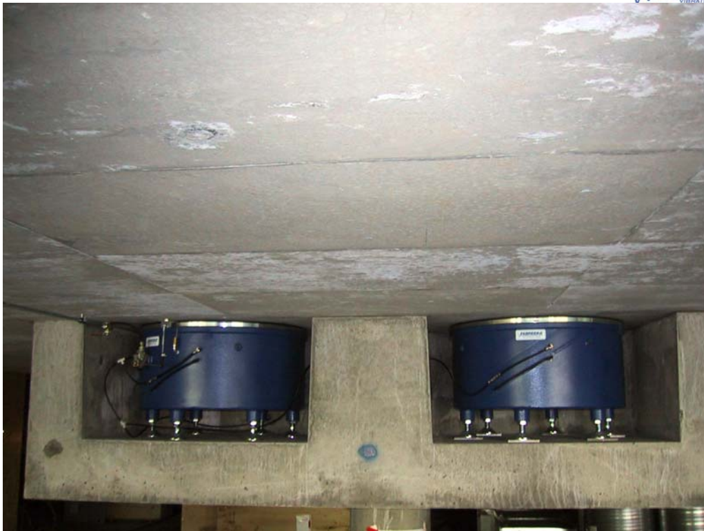
Sixty-six (66) PAL 1000 pneumatic isolators support the first and second floors of the wafer fabrication facility. Each isolator supports 120,000 lbs and has a vertical and horizontal natural frequency of 1.5 Hz.
