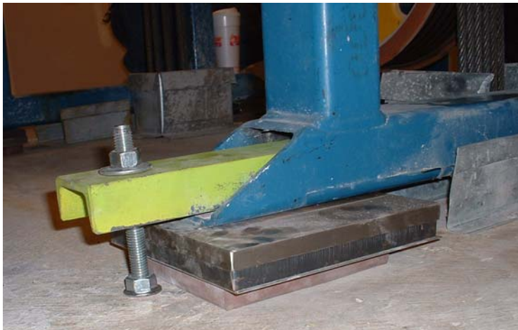
New FAB-EPM isolation material under elevator equipment.
