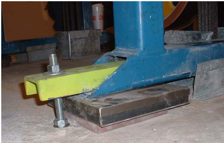
New FAB-EPM isolation material under elevator equipment.
