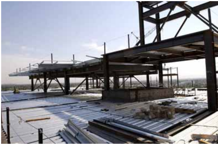
Early stages of building/heliport construction.
