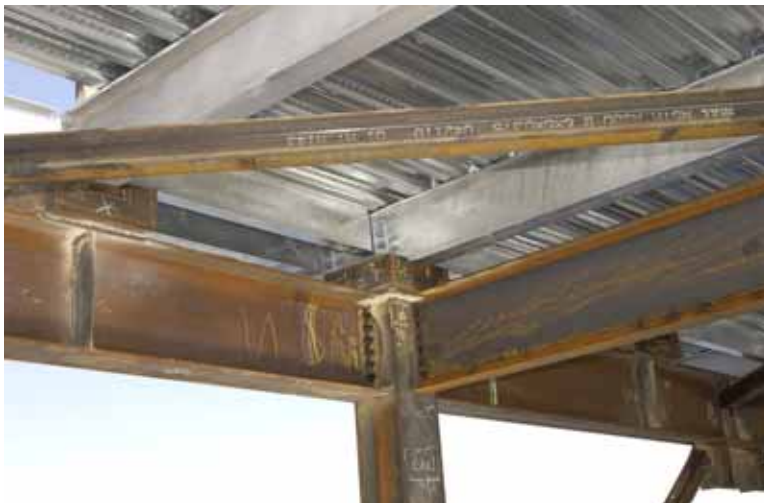
View of heliport on isolators "boxes" on the building support structure.
