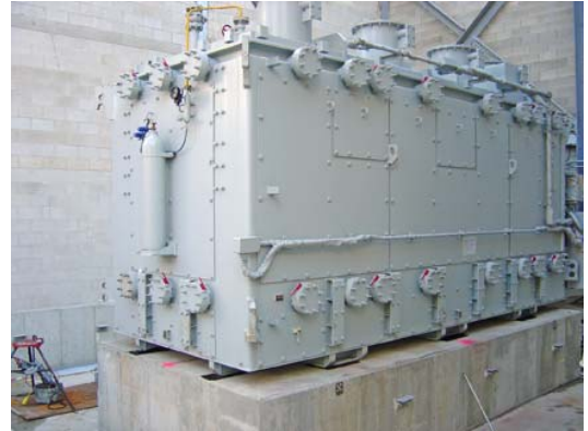
The transformer is lowered onto the Fabcel.
