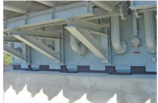
Fabcel pads are also used to support reactors.
